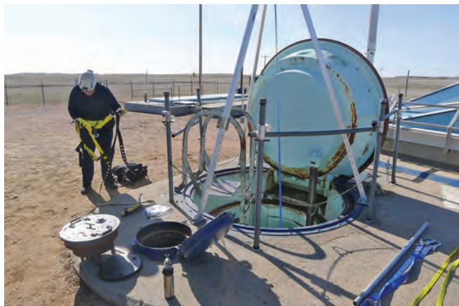
Personnel access hatch at D-9 LF. The hatch leads to a 25ft vertical shaft with a ladder for access
